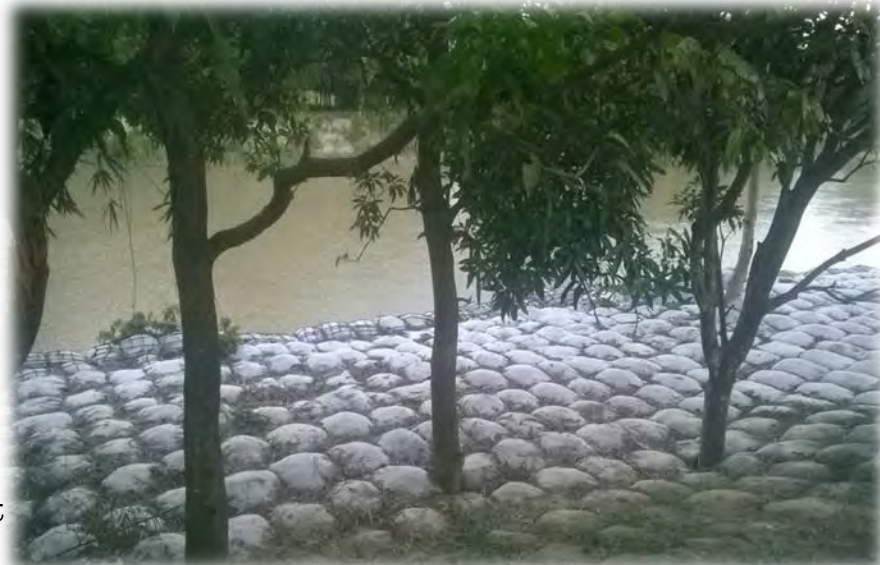
Khairi Mushehri 62 RD(left Kamla Embankment sand bagging)
