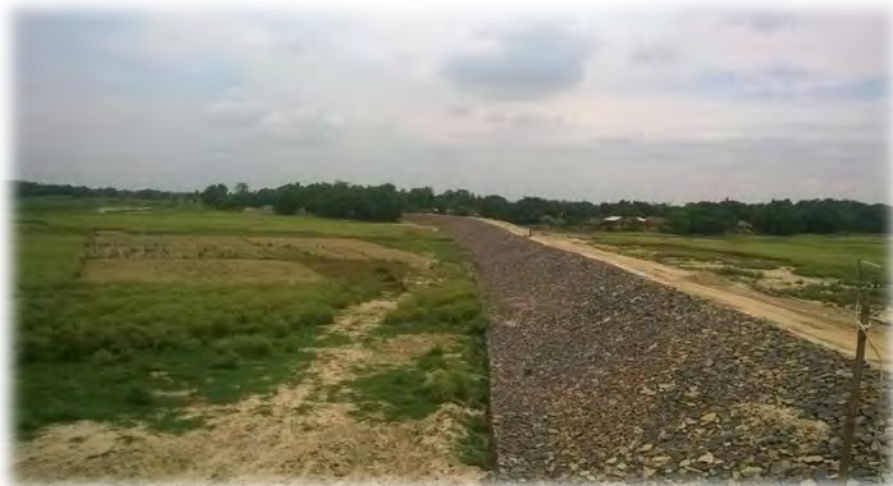
Stone pitching on Left Kamla Embankment at Fataki 64 Rd
